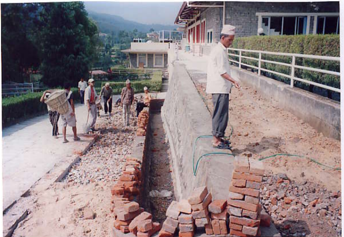
Back filling on Ramps in progress (View from North side)
