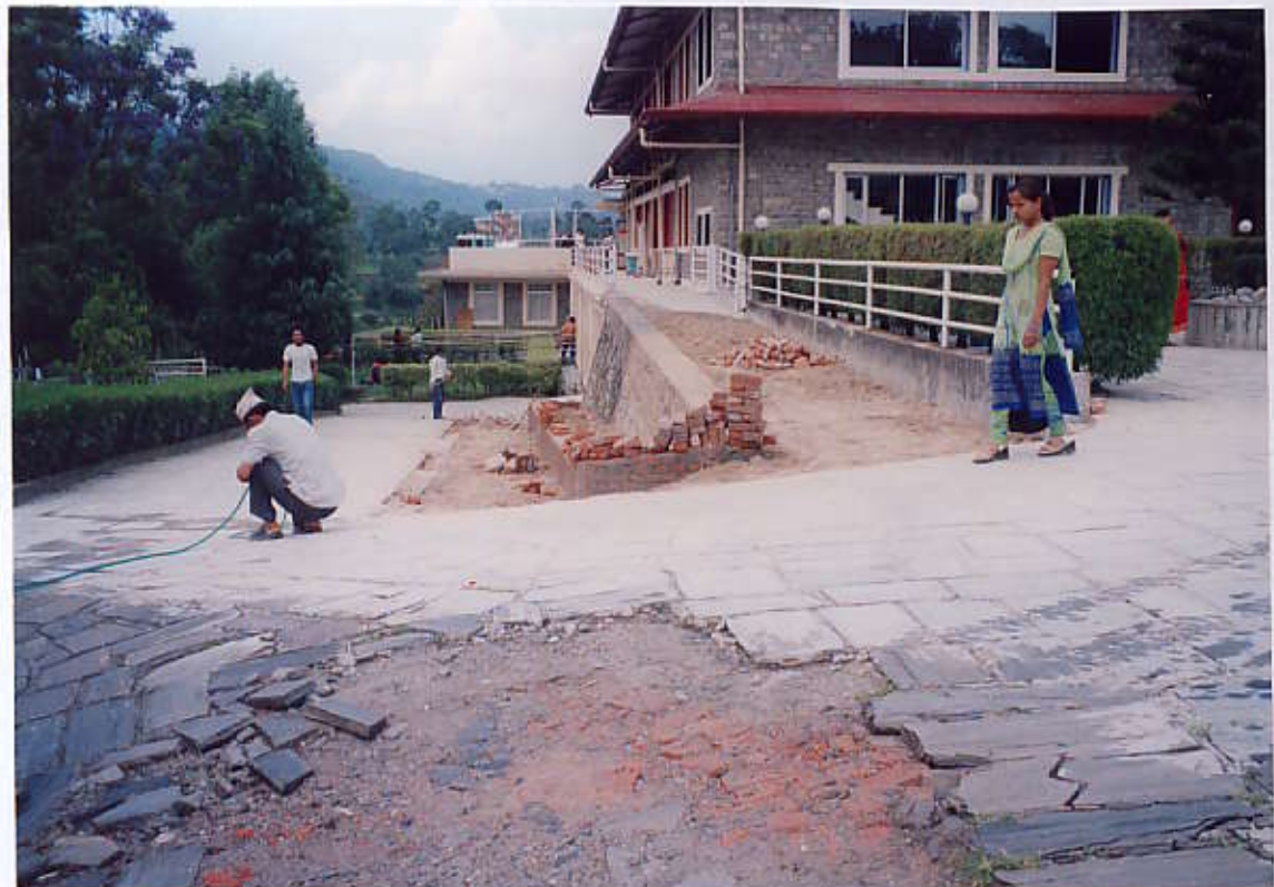
Back filled Ramps and existing Access Road (View from North side)
