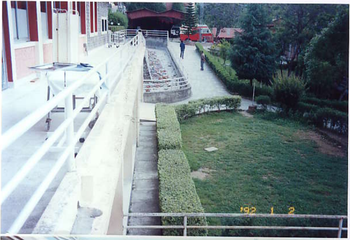
View of Lower Ramp, adjacent Access Road and Proposed Ambulance movement cum parking Area (Green Area) - (View from South Side)
