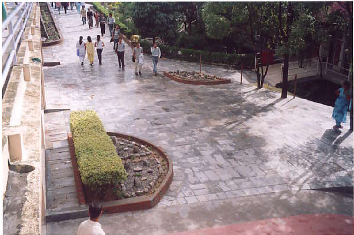
View of flag stone paved Ambulance movement & Parking Area (View from South side)
