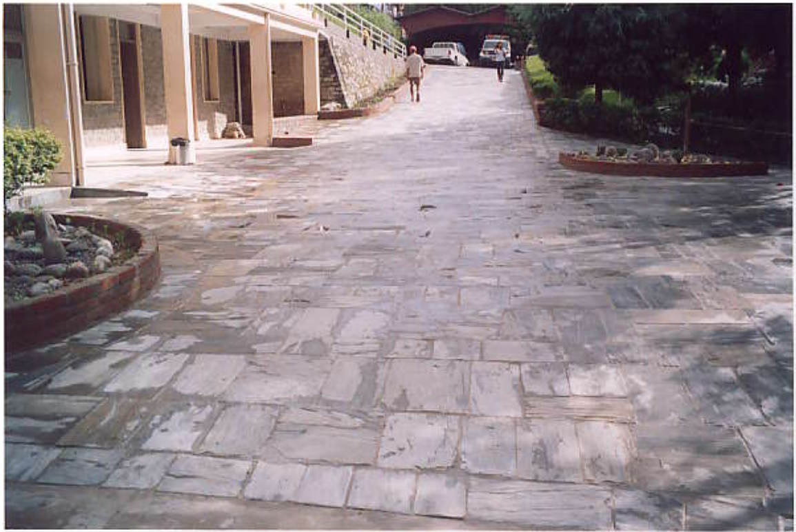
View of flag stone paved Access Road and Ambulance movement & Parking Area (View from South Side)
